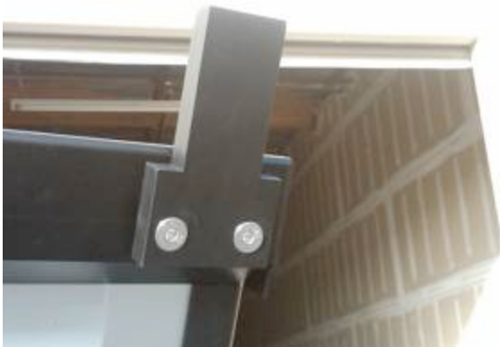
Bracket attaches to frame.
